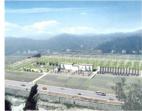
HVDC Converter Station > 6400 MW, Classic
